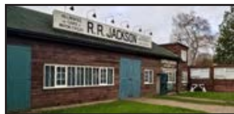
A period service garage
