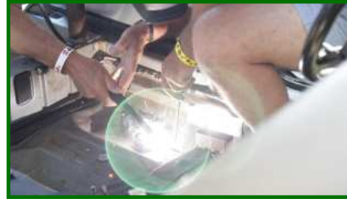
Welding in the pit (Photo by Buzz Hawes)
