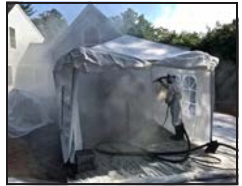
Nope, not a Covid-19 ward. This tent restricted the spread of all the dustless blasting particles.
